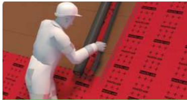
Sealing lateral overlaps with PAVATAPE 12 (ADB membrane).
