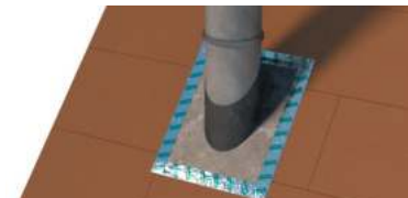
Seal the collar to the boards as explained on brick chimney. See Brick chimney sealing. Don't forget to prime!
