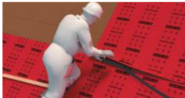
Self-sealing longitudinal overlaps (ADB membrane).
